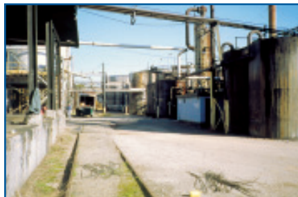
Chemical plant prior to demolition.
