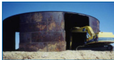
Tank contents removal.
