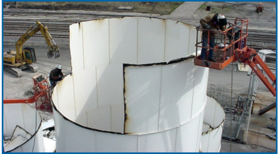
Silo demolition and hot work.
