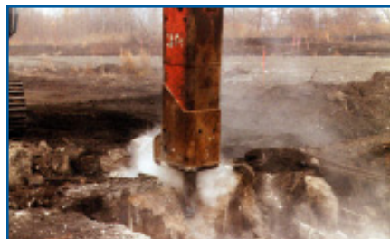
Concrete demolition work.
