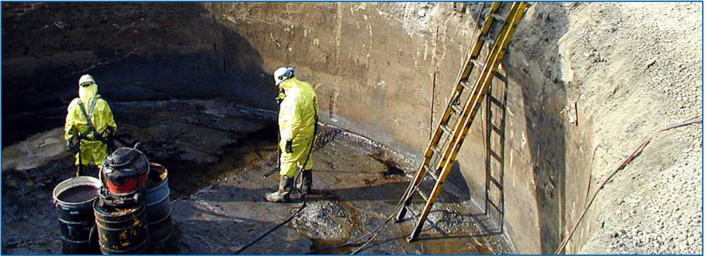
Gas Holder base cleaning and inspection.
